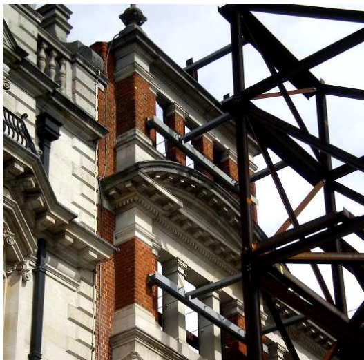
Retained façade of Audit House
