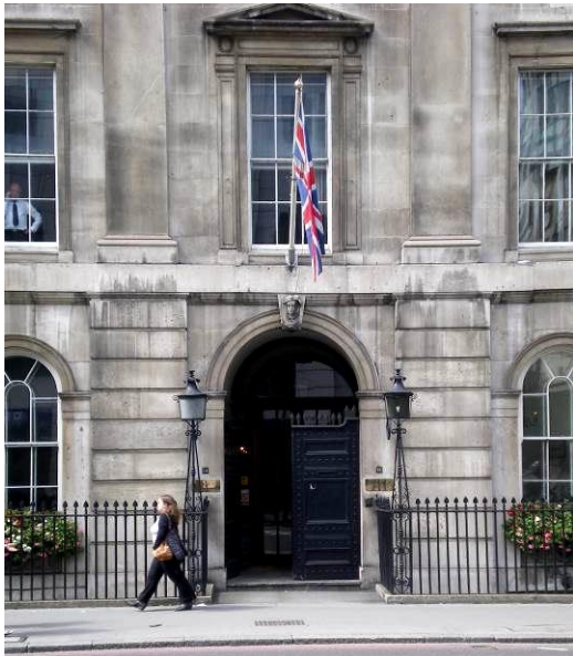
14 & 19 New Bridge Street
