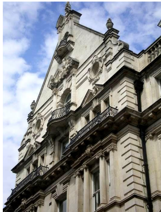
Telephone House (detail)
